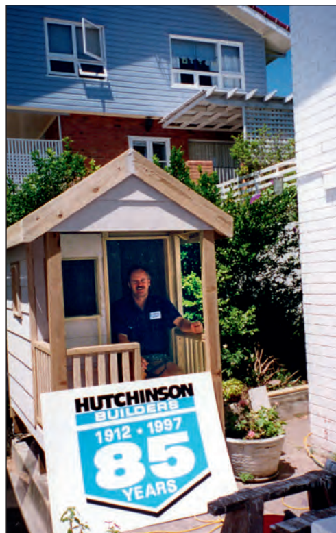
HUTCHIES has hung the sign on some unusual projects in the past 88 years, but this one takes some beating. Kevin Hall, is shown putting the finishing touches to a cubby house at Susan Blue's residence.
